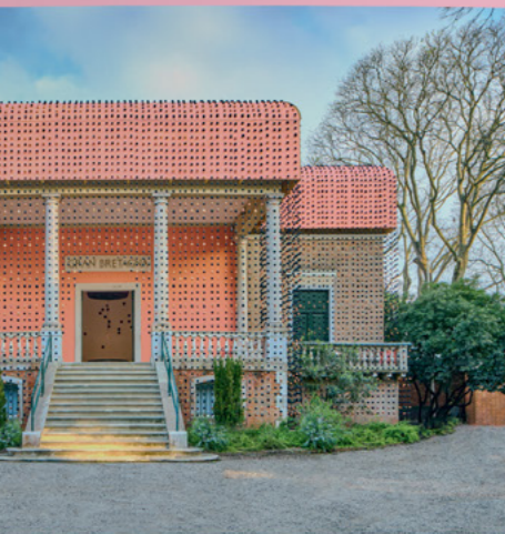
g Cave_Bureau (see British Pavilion at the aces the entangled struction, asking bilities embedded g the façade is made ndian soil - materials displacement.
